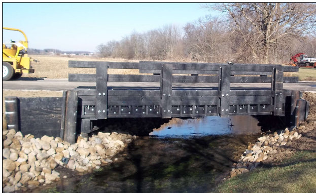
Bridge 174-0.56 over the Onion Ditch
